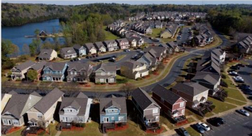
Emmons Roofing and Siding replaced the roofs on all 288 homes and three clubhouses at The Cottages at Lake Tamaha, a housing complex in Tuscaloosa, Alabama.
